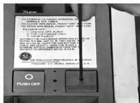
Activating the switch closing mechanism through the hole in the Hidden "ON" Button
