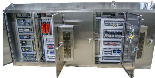
This panel was built for process and motor control of a bottling line in the food industry. ECT provided designed assistance and fabricated the panel.
